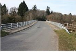
Old Exeter Road IMG_3484
