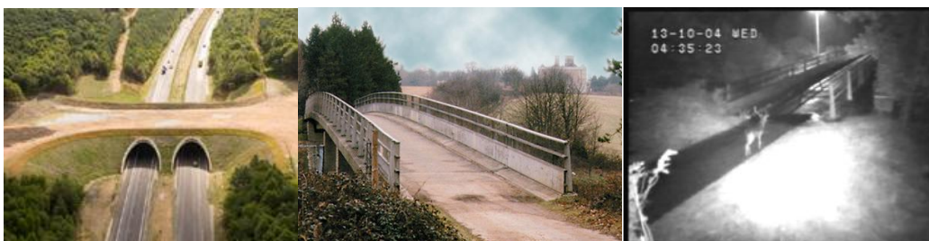
Photos 4, 5 and 6: A large green habitat bridge in Switzerland (left) and a narrow joint use bridge with concrete substrate across M25 nr London (centre & right): each structure was designed for a quite different set of aims but both are regularly used by deer.
