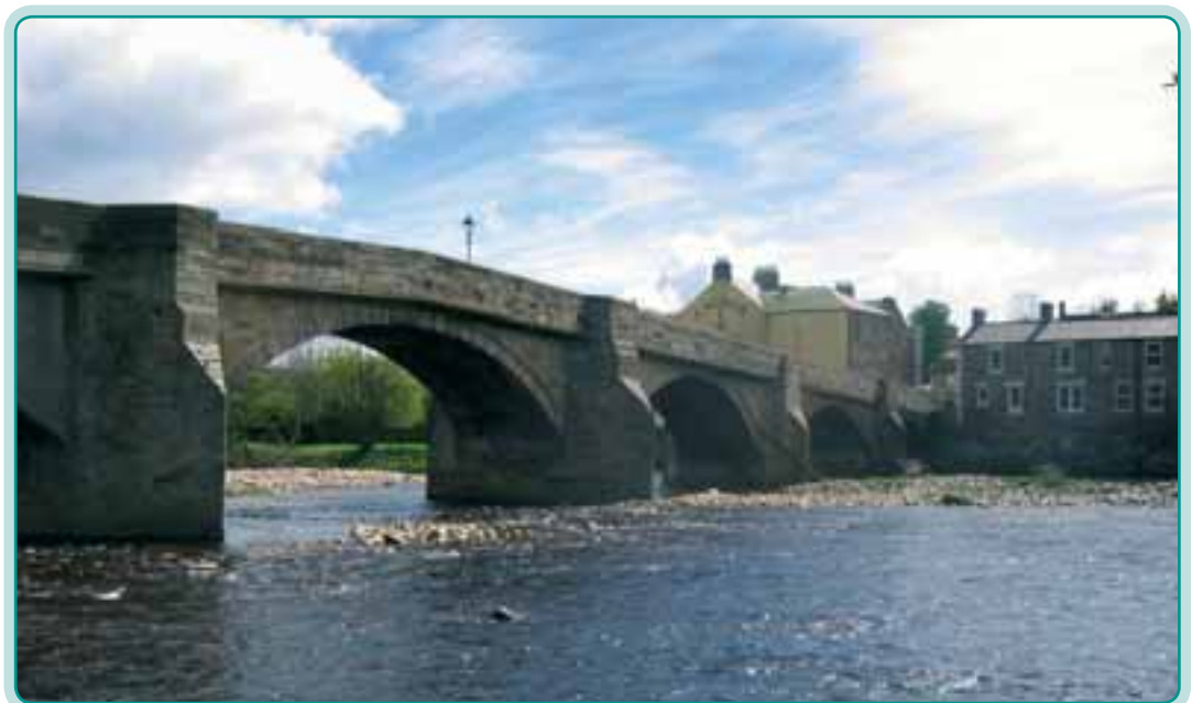
The historic bridge over the River South Tyne.
