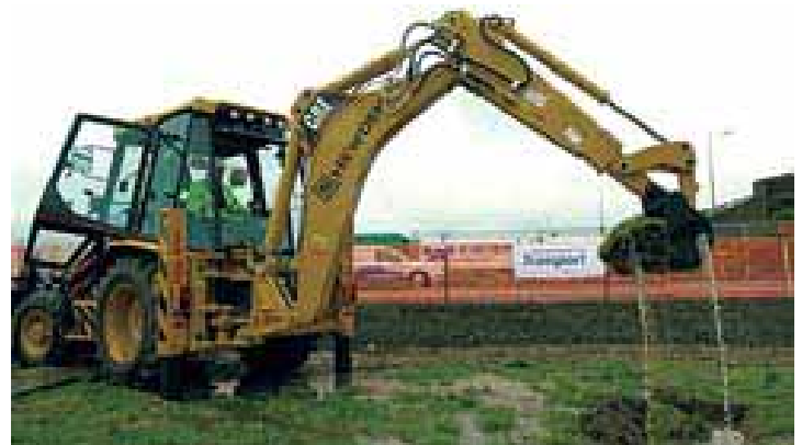
Roads Minister, David Jamieson starts excavation for new bridge
