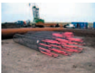
Cages used to reinforce concrete piles
