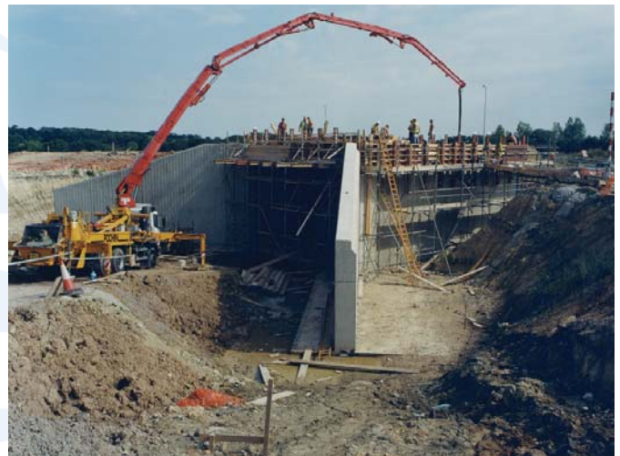
Pouring Concrete on Baytree Lane underpass by Cophall Roundabout
