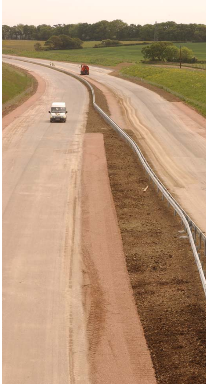
A27 Bypass route nearing completion
