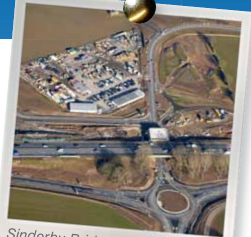
Sinderby Bridge and the site compound
