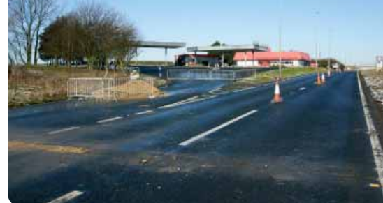
Former Rainton Services site - now closed
