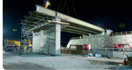
Overnight beam placing at Londonderry
