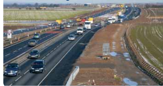
Looking from Baldersby Bridge to Rainton Bridge on the horizon
