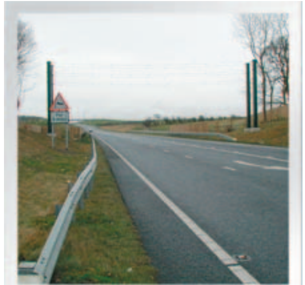
Example of a Bat Bridge.
