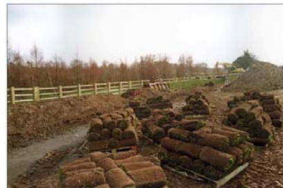
Mitigation Measures Hedgebank :- under construction
