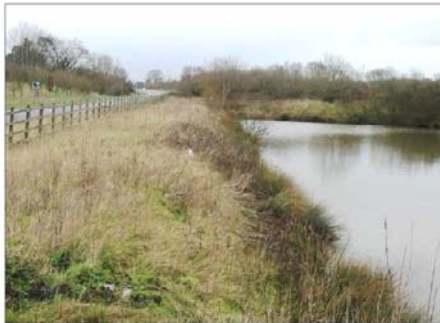
Drainage Attenuation Lagoon
