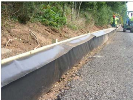
New reptile fence on M4 Motorway
