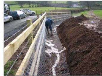
Mitigation Measures :- Badger proof fencing being installed
