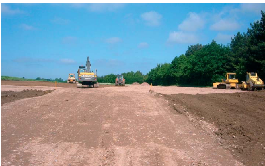
Preparation for Site Compound
