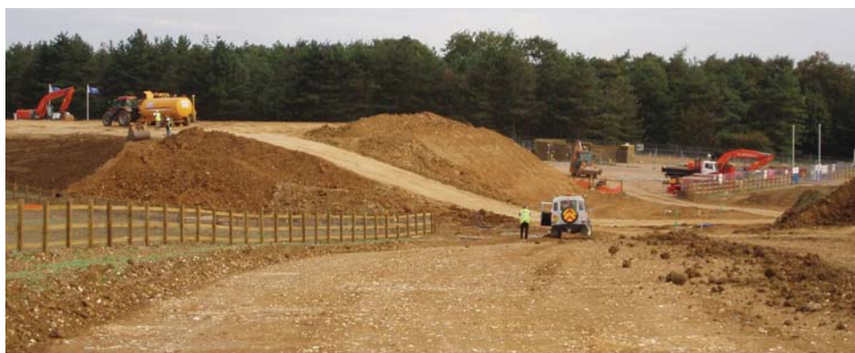
Construction of the new Haughley Road
