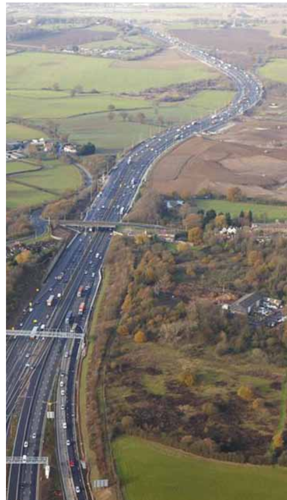
From above the slip roads at junction 23 towards junction 22 – South Mimms bund earthworks on the right
