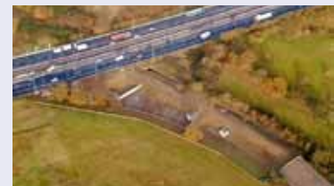
Pond 21 after construction
