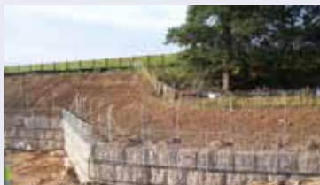
Use of gabion walls protects oak trees and retains the pond's volume
