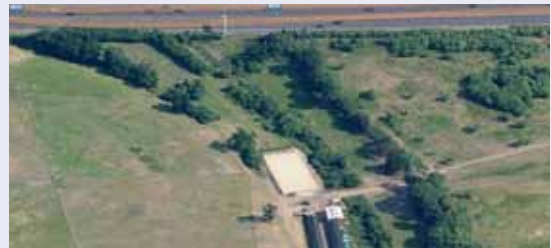
Pond 21 area before construction
