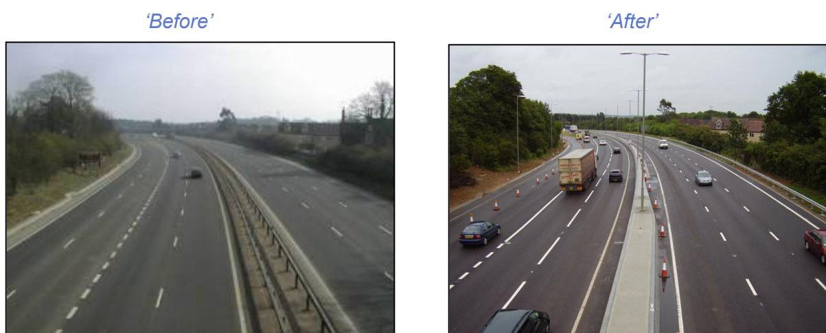
Figure 2.1 – Pre and Post Scheme Opening Safety Barrier and Lighting
