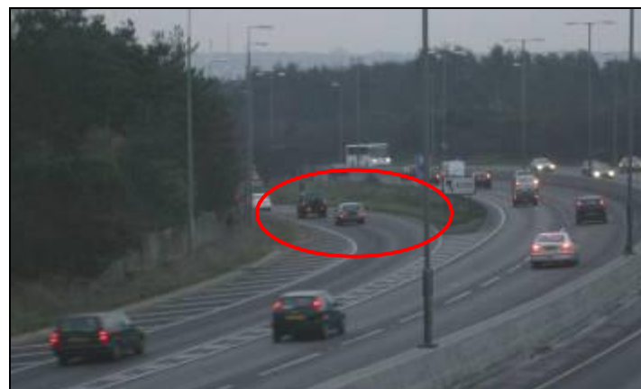
Figure 2.6 – Remedial Measures Implemented at J27 Off-slip
