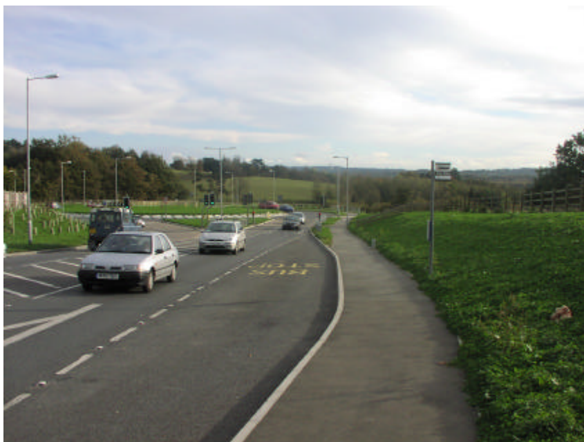
Figure 5.7 – New Bus Stop on West Side of A21
