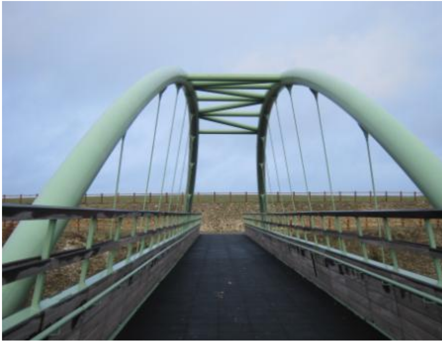
Figure 7.3 – Rubber Tiles on Bridge Deck to Reduce Noise
