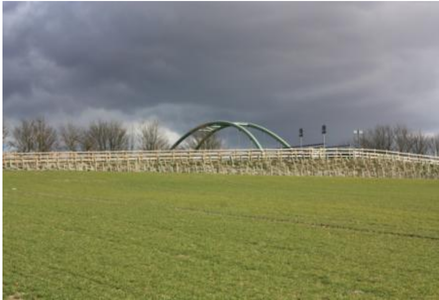
Figure 7.2 – Bridge Structure Visible Over Top of the Cutting
