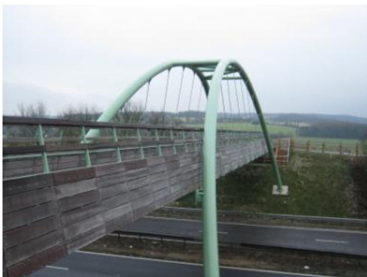
Figure 2.2 – Bridge Structure with Timber Cladding
