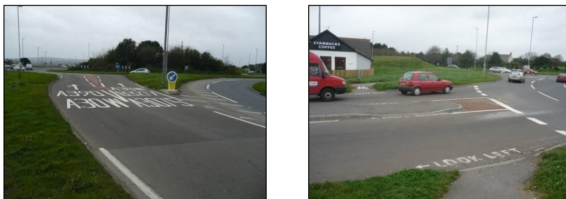
Figure 2.2 - Subsidiary islands on the A30 and A390 entries to improve deflection on entry 1 .
