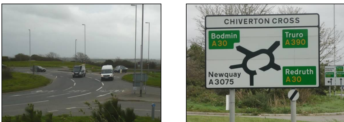
Figure 2.1 – Spiral type road markings to delineate traffic lanes on the circulatory carriageway, together with additional direction signing on the approaches, to assist lane discipline
