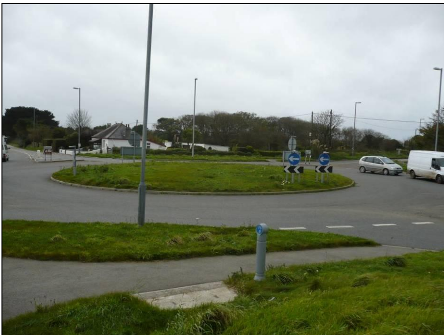
Figure 2.4 - New subsidiary roundabout linking the B3277 to St Agnes and road to Blackwater and replacement link to the main roundabout to reduce number of arms.
