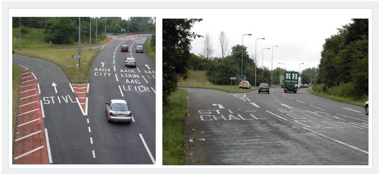
Figure 2.4 - Lane Markings 'before' (Right) and 'After' (Left) Opening
