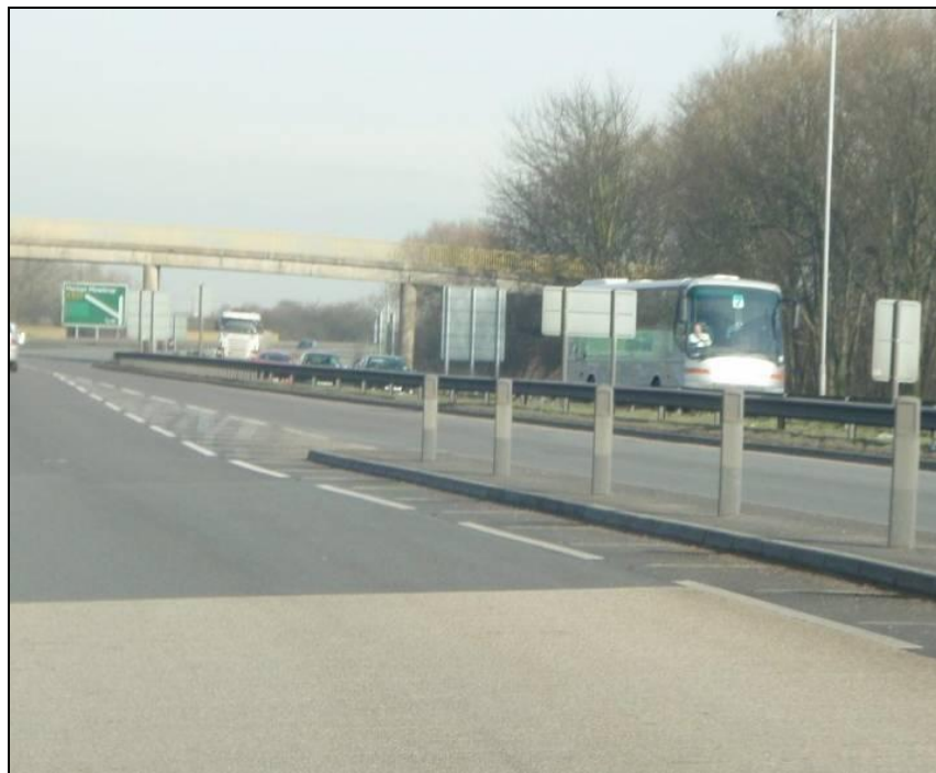
Figure 2.3 – Reflective Marker Posts on A46 (N) Arm
