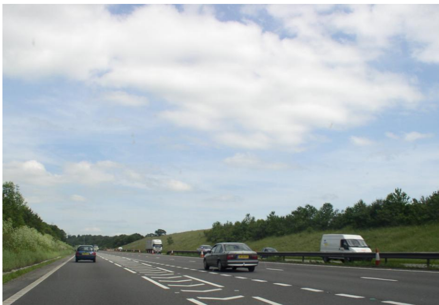
Figure 1.3 – Ghost Island merge from the A483 (N) slip road to the A55
