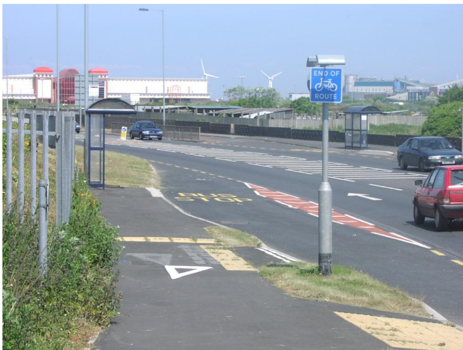
Figure 5.3 - An Example of the New Cycle and Pedestrian Facilities at Northside
