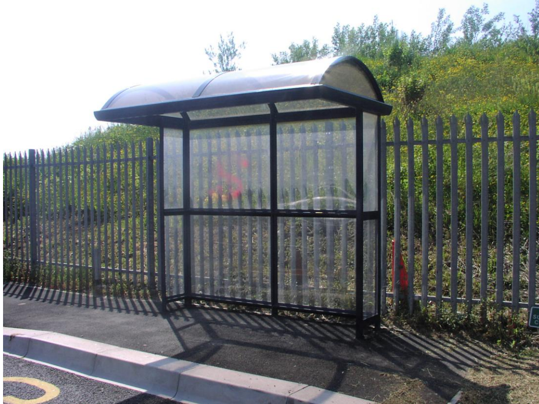
Figure 5.4 – The New Bus Bay on the A596
