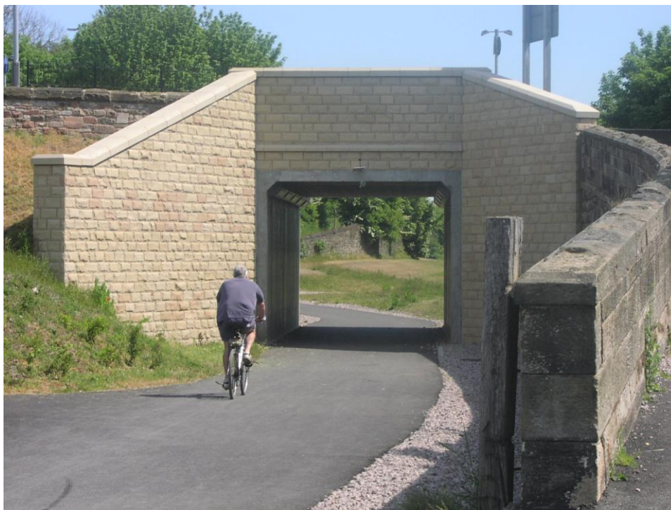
C4: Underpass at Calva Brow roundabout
