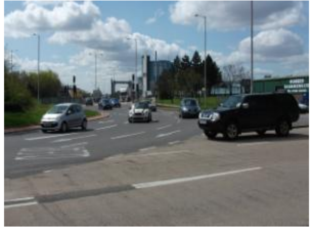
After Scheme Opening (Looking West)
