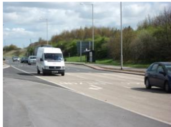
After Opening (Looking East)
