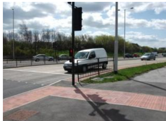
After Scheme Opening (Looking West)
