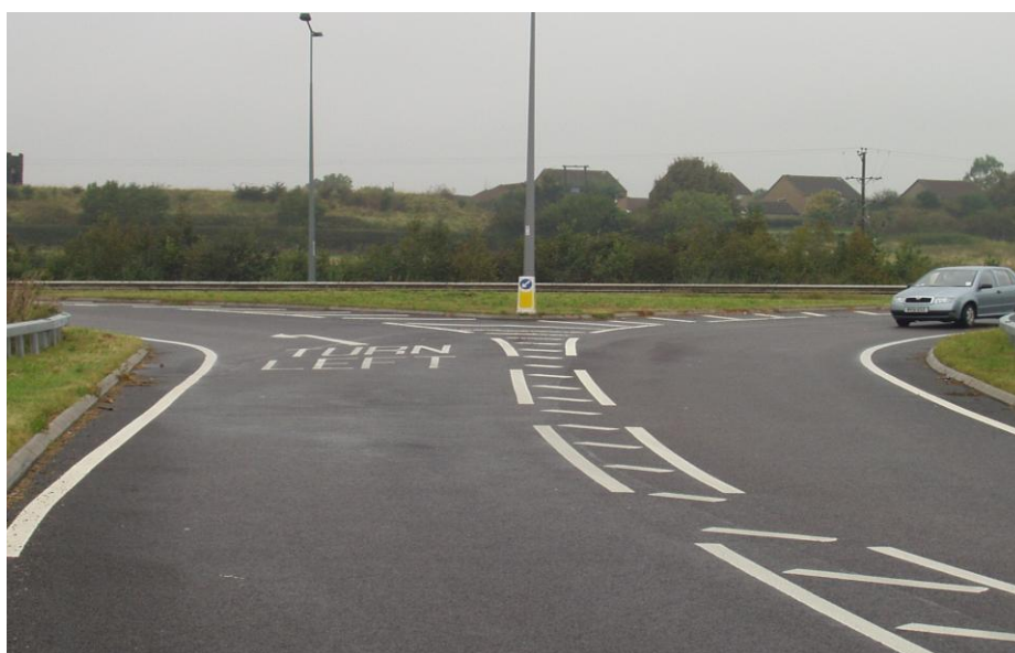
Figure 1.1 – New Merge/Diverge on the A66 at Sadberge (WB Carriageway)
