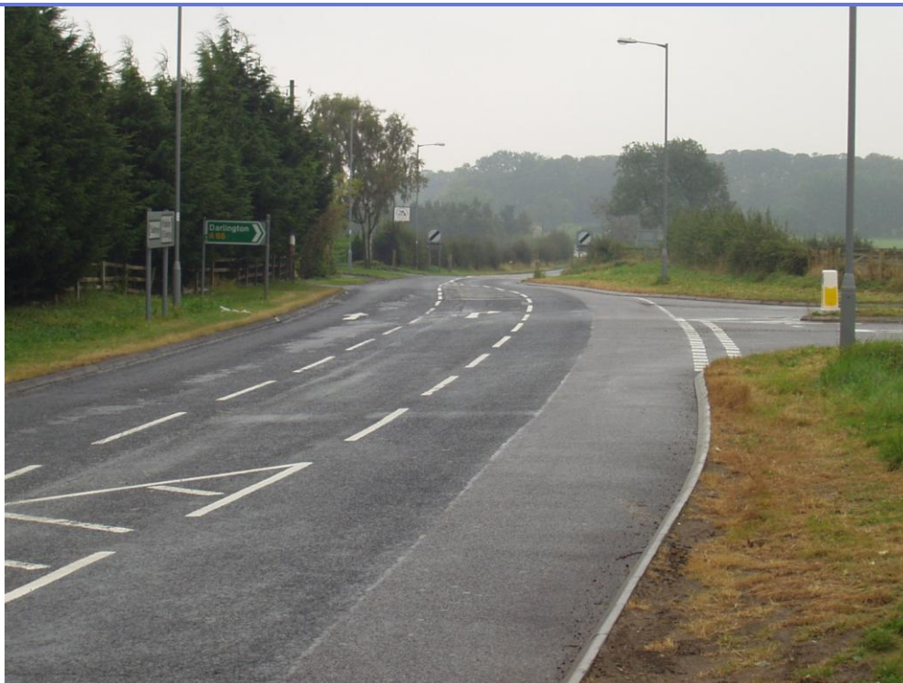
Figure A3 – New Priority Junction on Local Road Network at Middleton Road
