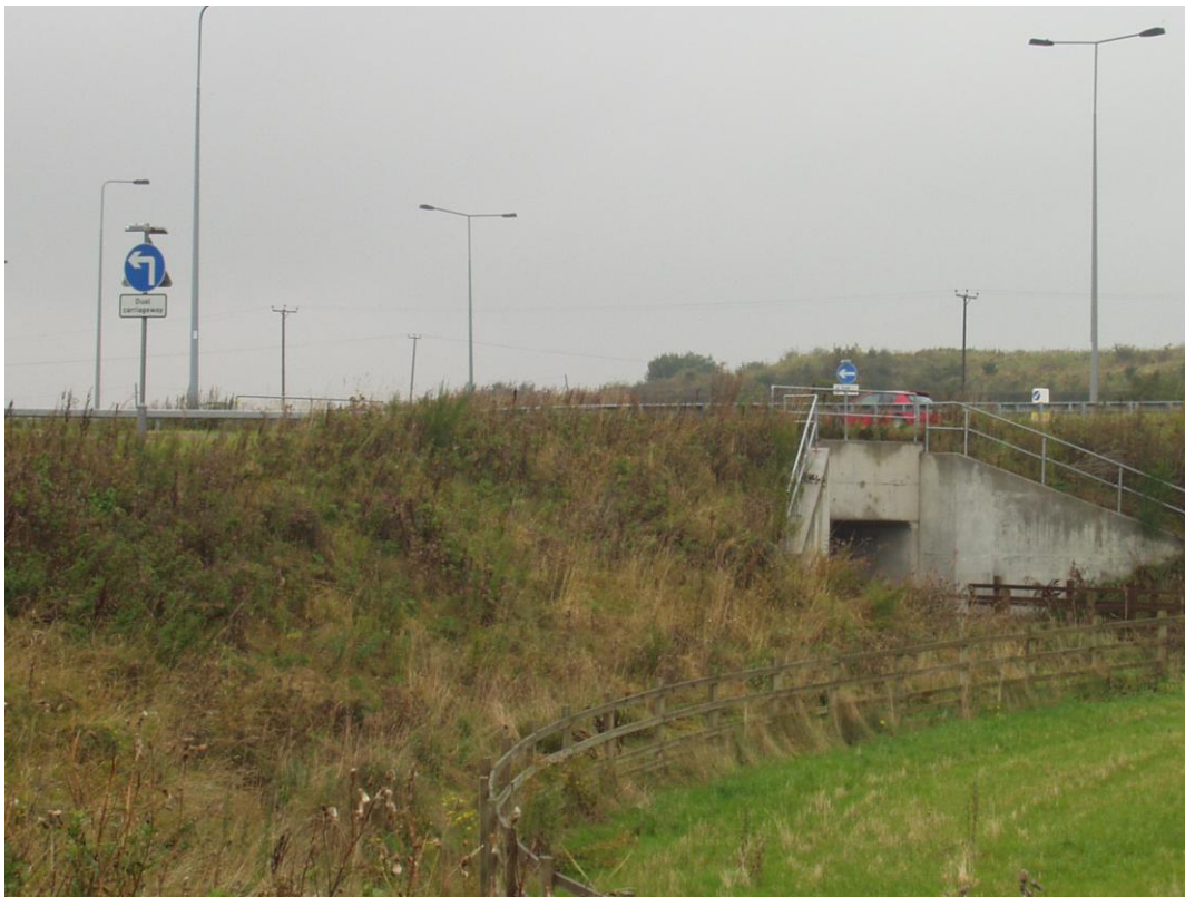
Figure 5.3 – Photo of Scheme and New Agricultural Underpass
