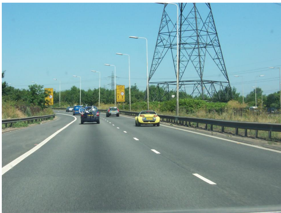
Figure 1-1 – Reinstated two lane slip from A406 north to M11 north
