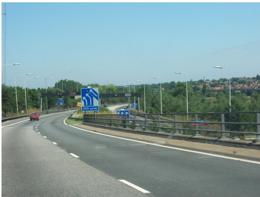
Figure 5-1 – A406 Northbound to M11 Northbound Merge
