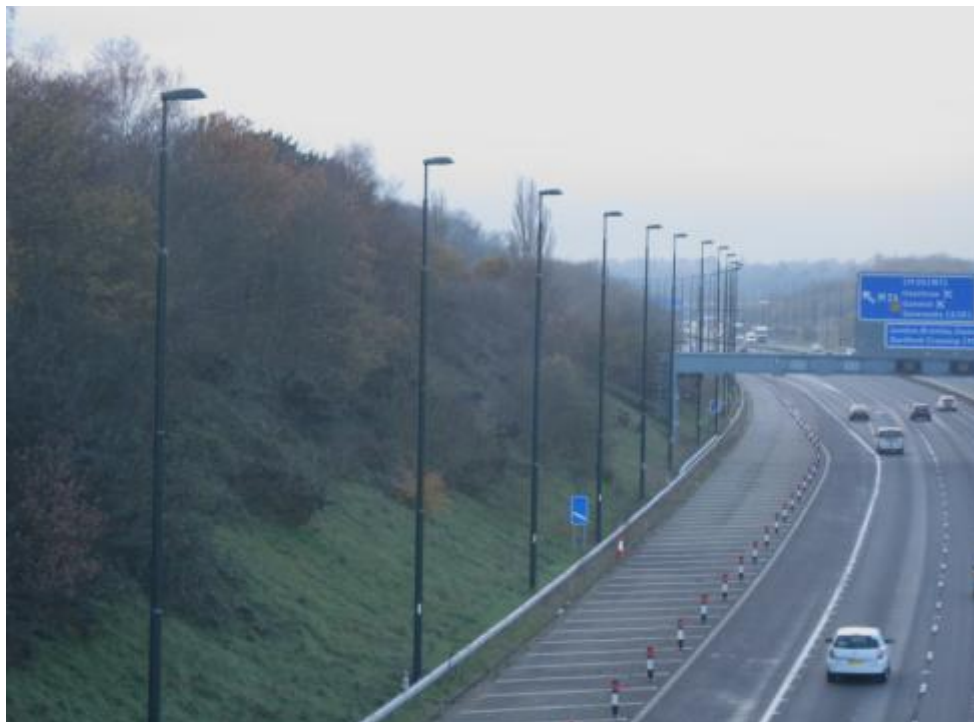
Figure 2.3 – Lamp Columns Painted Green
