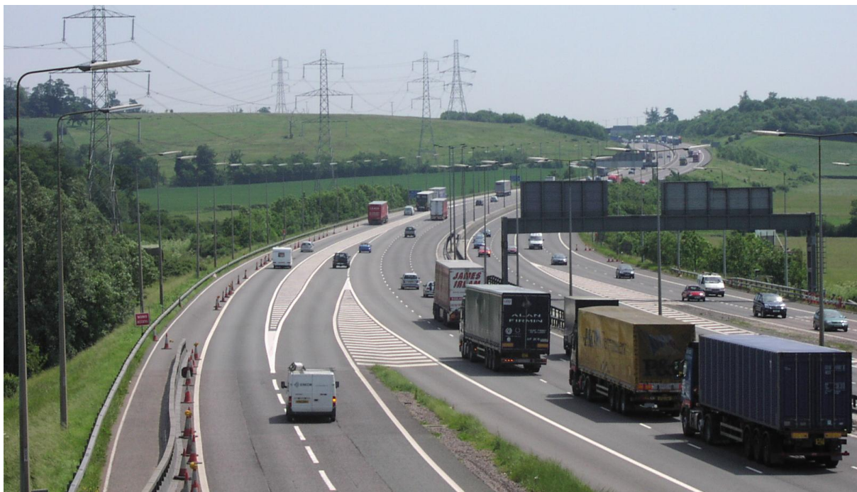
Figure 1.3 - Photograph of climbing lane site 4
