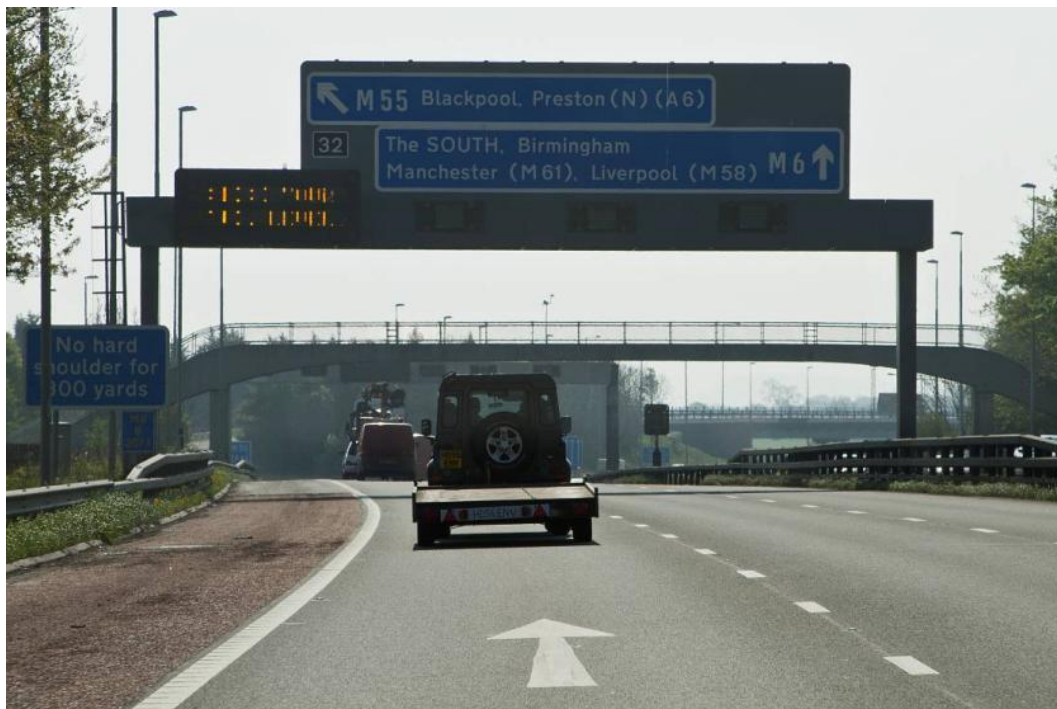
Figure 2.4 – Example of new gantry signing on approach to Junction 32
