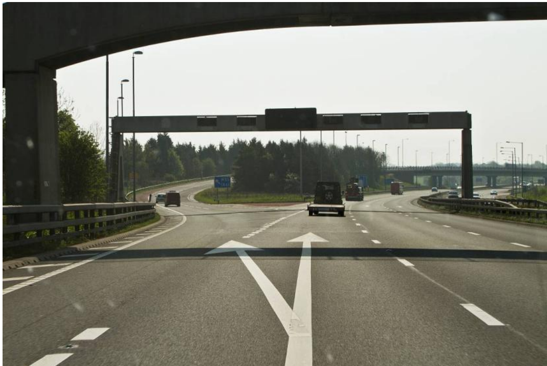
Figure 2.6 – New J32 SB diverge and 3 lane through junction layout
