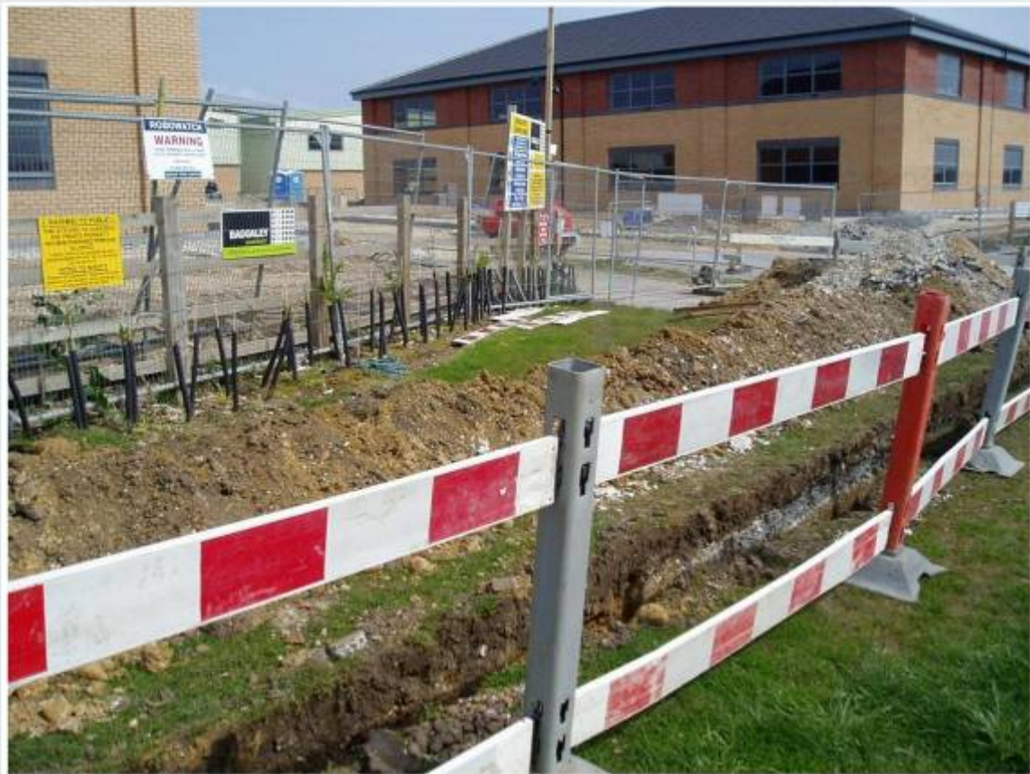
Figure 2 – Development Under Construction
