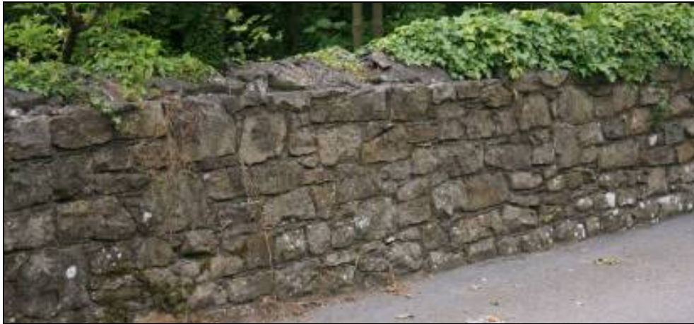
Figure G.5 - Existing walls near Scale Beck crossing
