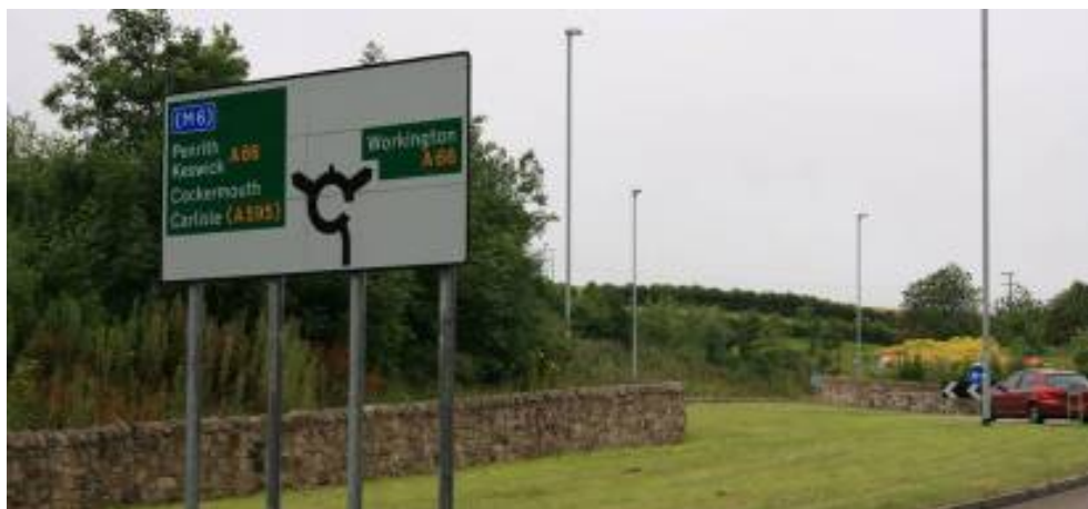
Figure G.19 - Full cut off lighting and signage at the western roundabout
