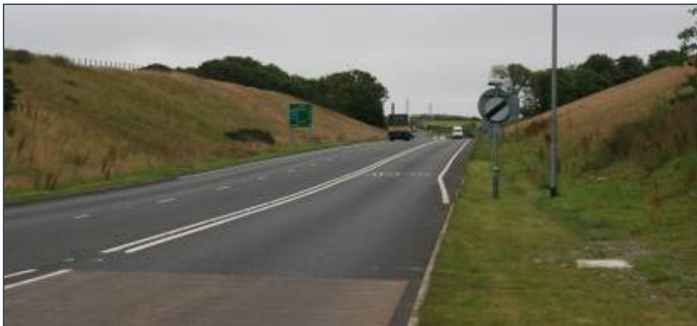
Figure G.12 - Deep cutting through Upper Park reduces impact of the road
