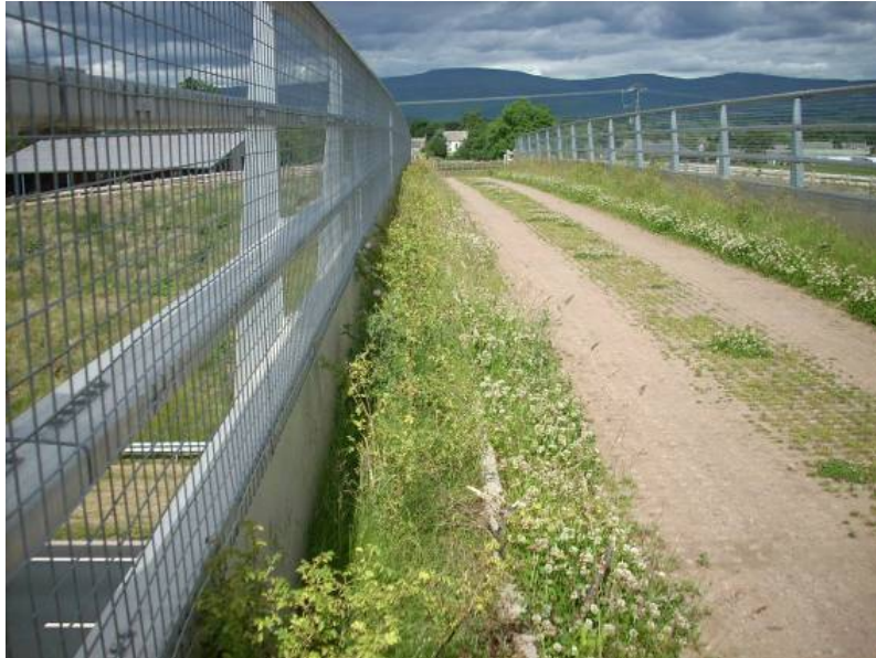
Figure C.10 – Green bridge carrying the bridleway over the bypass
