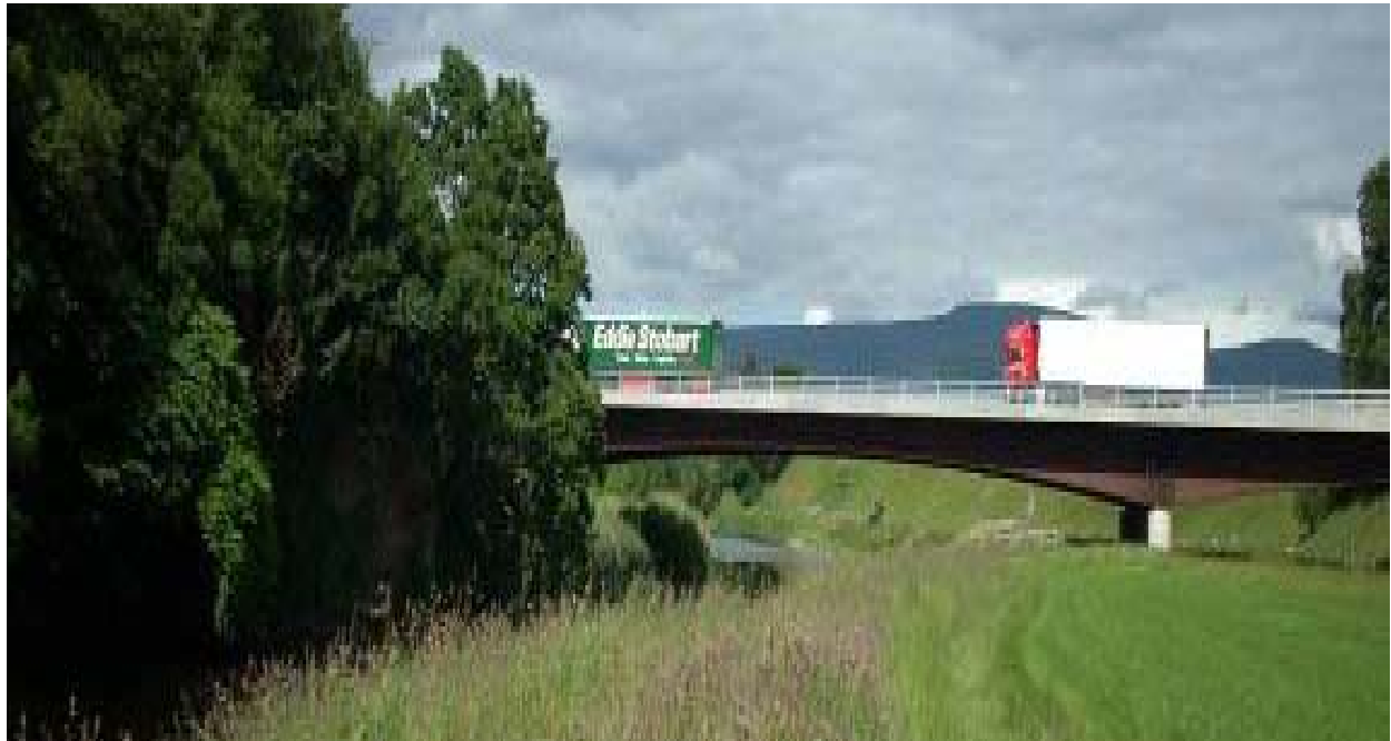
Figure C.7 – The new bridge crossing the River Eden is constructed from steel and concrete with a metal balustrade. The view from the PROW along the riverbank has been adversely affected
