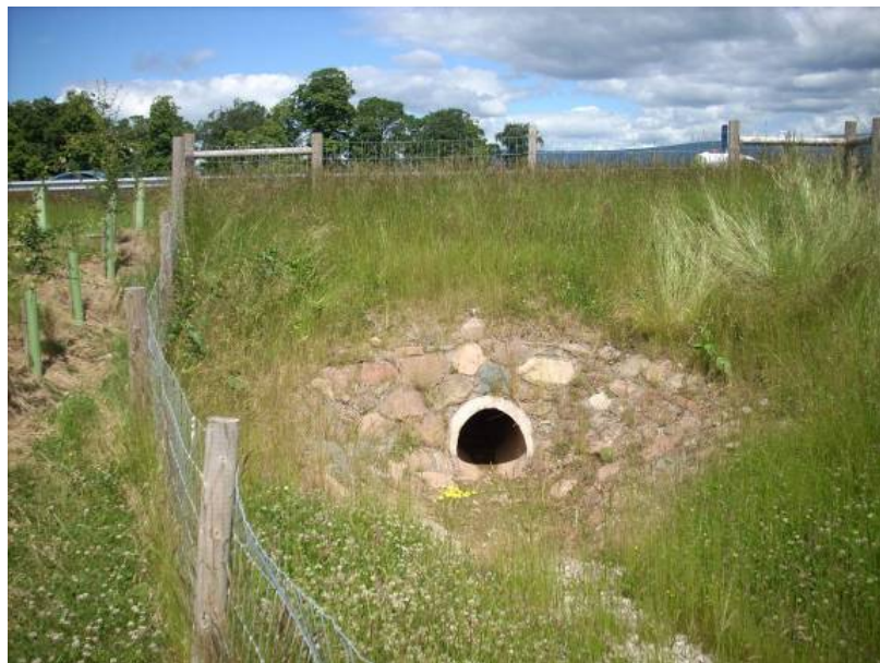
Figure C.8 – Mammal crossing near Cliburn Road junction
