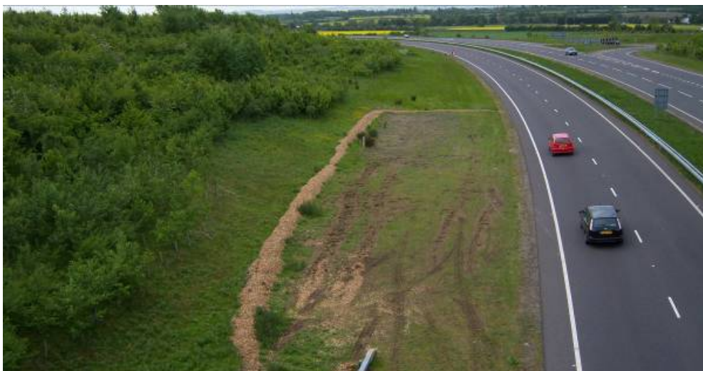
Figure B.10 French drain on southbound carriageway near Highfield Road bridge
