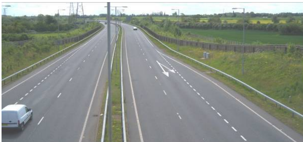
Figure B.1 Environmental barriers both sides of the carriageway southbound from Oakley Road junction over-bridge
