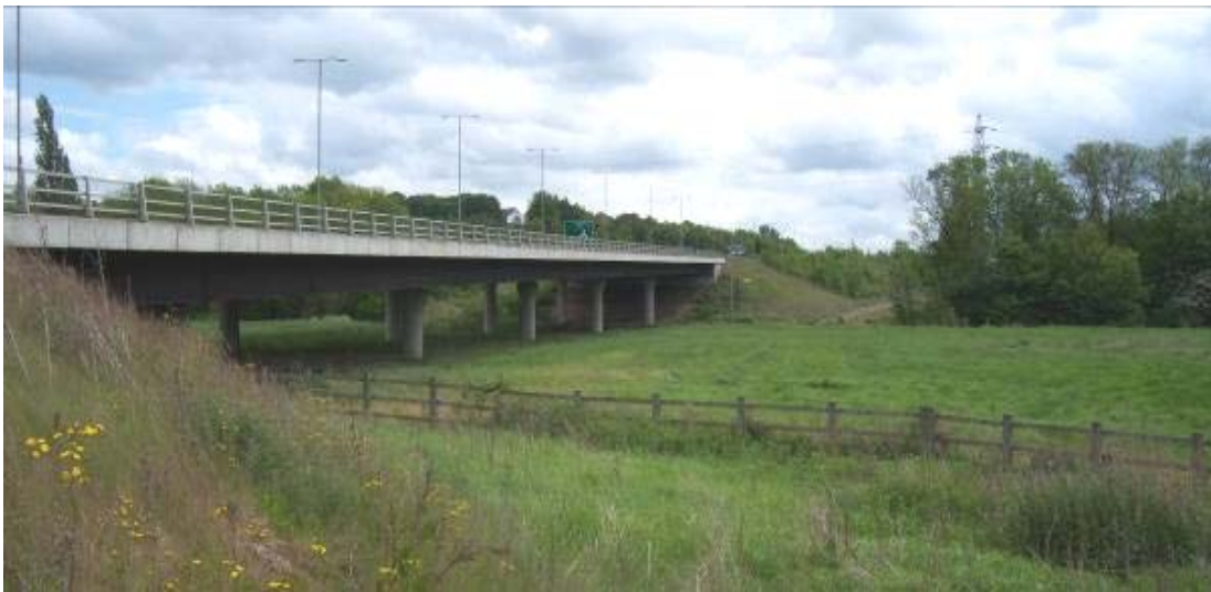
Figure B.11 South Ouse crossing illustrating low profile bridge to minimise visual impact within the floodplain
