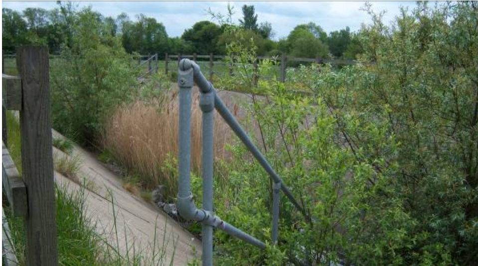
Figure B.8 Spillage containment basin north of south Ouse bridge
