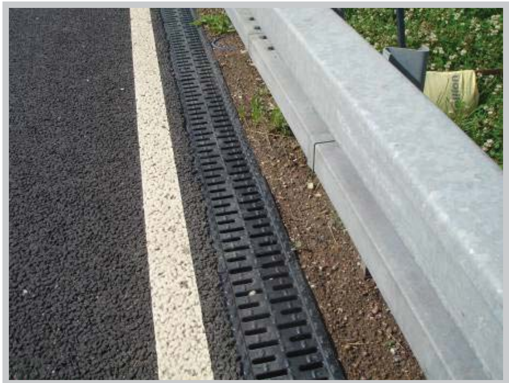
Figure I.20 - Edge of highway gully located on the northbound carriageway
