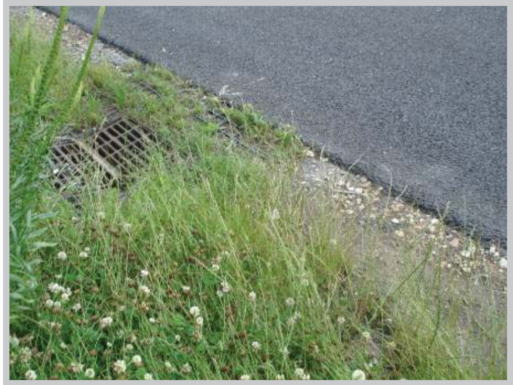
Figure I.21 - Filter drain located on the edge of the carriageway
