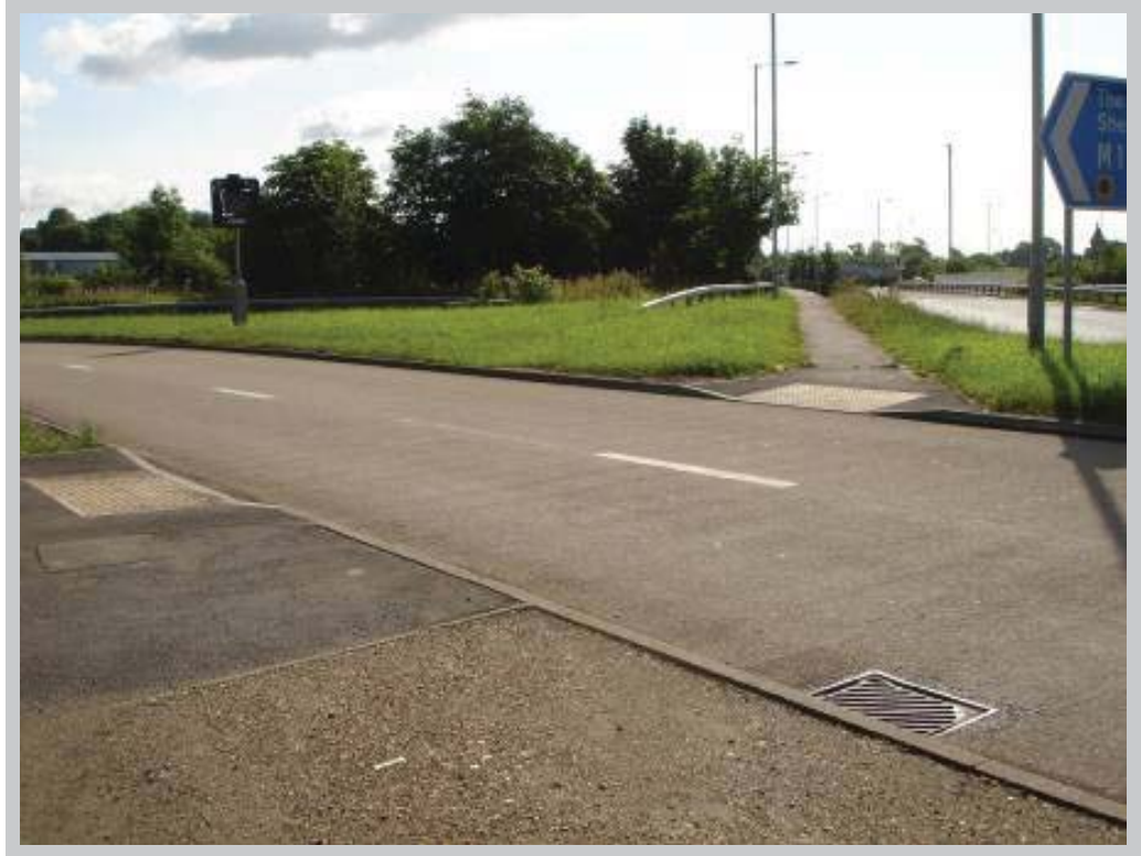
Figure I.13 - Dropped kerb at pedestrian crossing point on the roundabout at Junction 31
