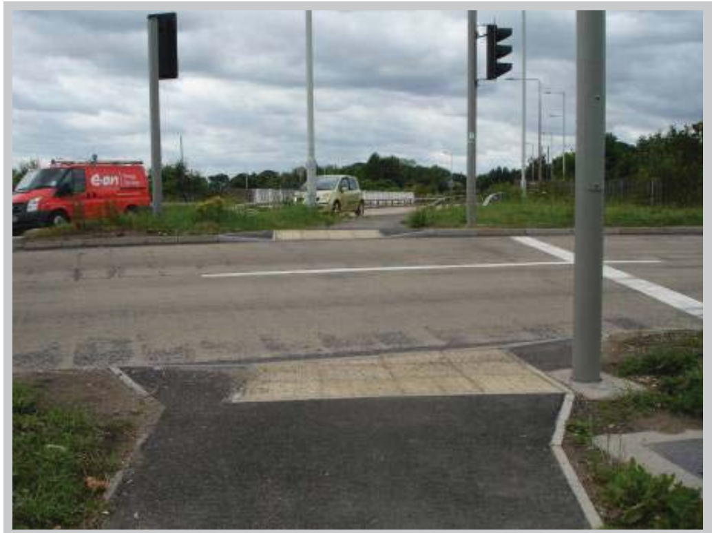
Figure I.24 - Dropped kerb at pedestrian crossing point on the roundabout at Junction 31
