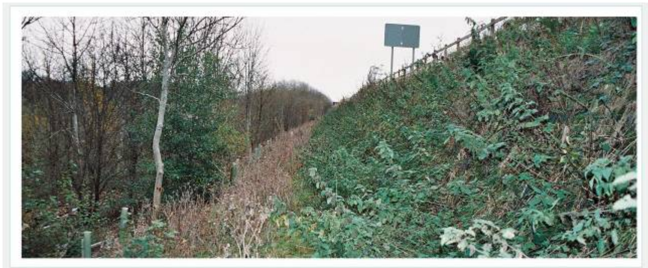
Figure 5.2 – Reinforced earth slope at top of embankment slope
