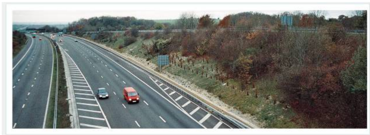
Figure 5.3 – Calcareous soil area above retaining wall allowed to re-colonise naturally
