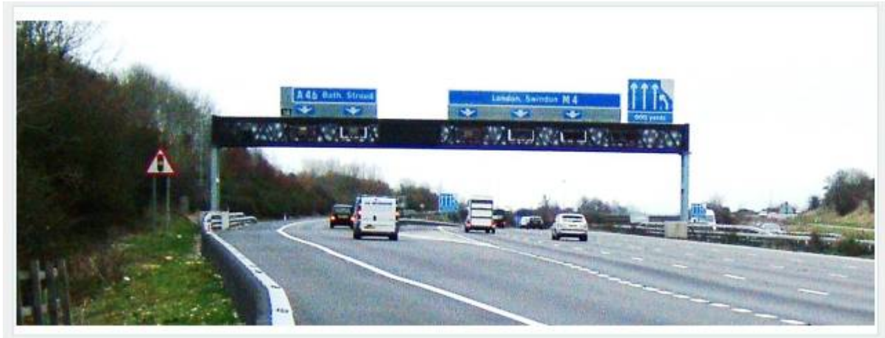
Figure 5.9 – Gantry 3 near the Junction 18 off slip
