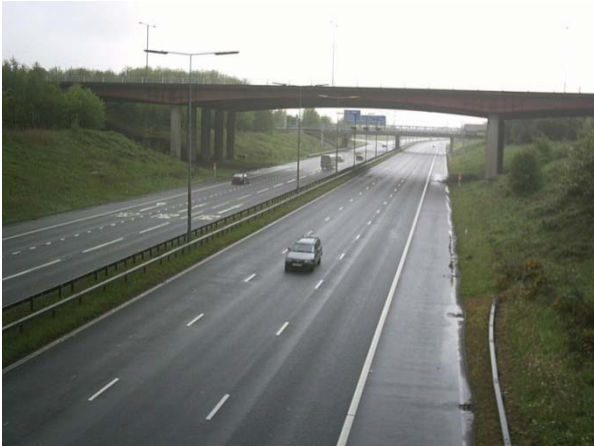
Figure 1.4 – M62 & M57 Overbridge
