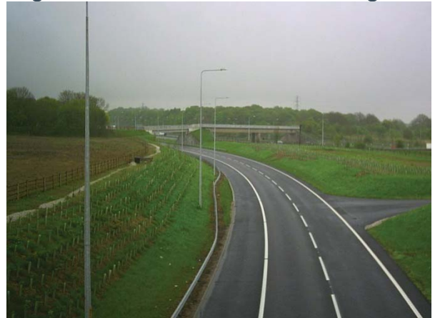
Figure 1.7 – New Link A & Potters Pits Bridge with New Extension to Left
