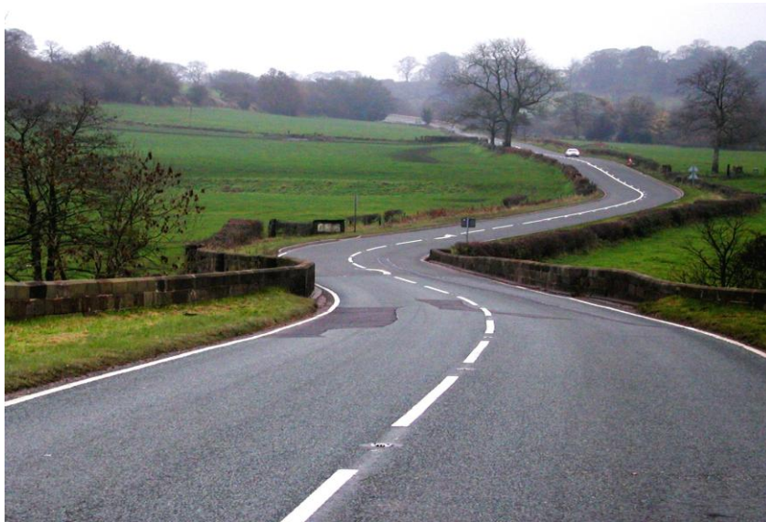
Figure 1.2 – Bridge Over River Dene BEFORE Safety Scheme
