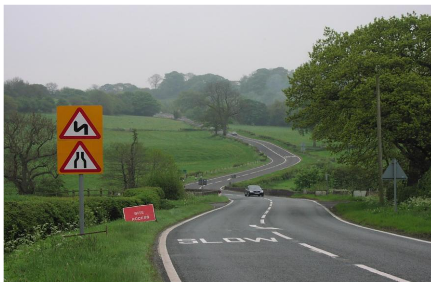
Figure 1.3 – Bridge Over River AFTER Safety Scheme
